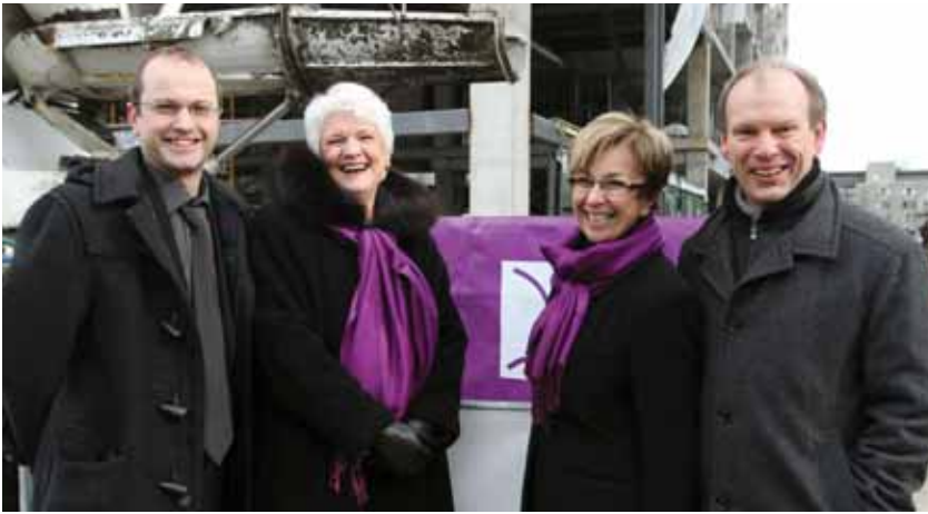
Construction milestone: When the highest point of the new Bell Gateway Building was reached in January, the CAMH community celebrated the building's final concrete pour with a traditional "topping off" ceremony directed by the Honourable Liz Sandals (second left), Parliamentary Assistant to the Minister of Health and Long-Term Care, shown alongside city councillor Michael Layton (far left), CAMH CEO Dr. Catherine Zahn and Matt Ainley of Carillion Canada.
